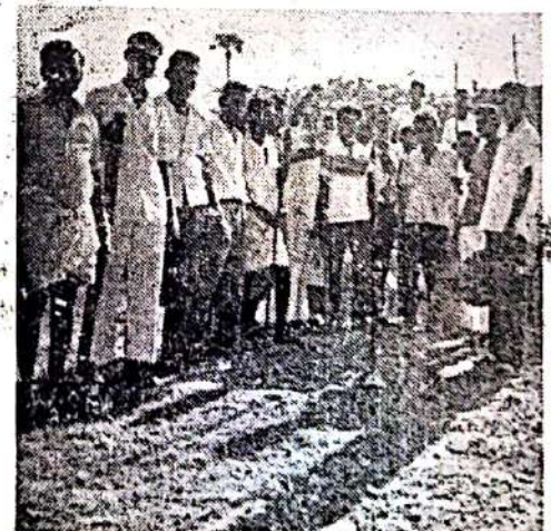
Trainees at cleaning work
